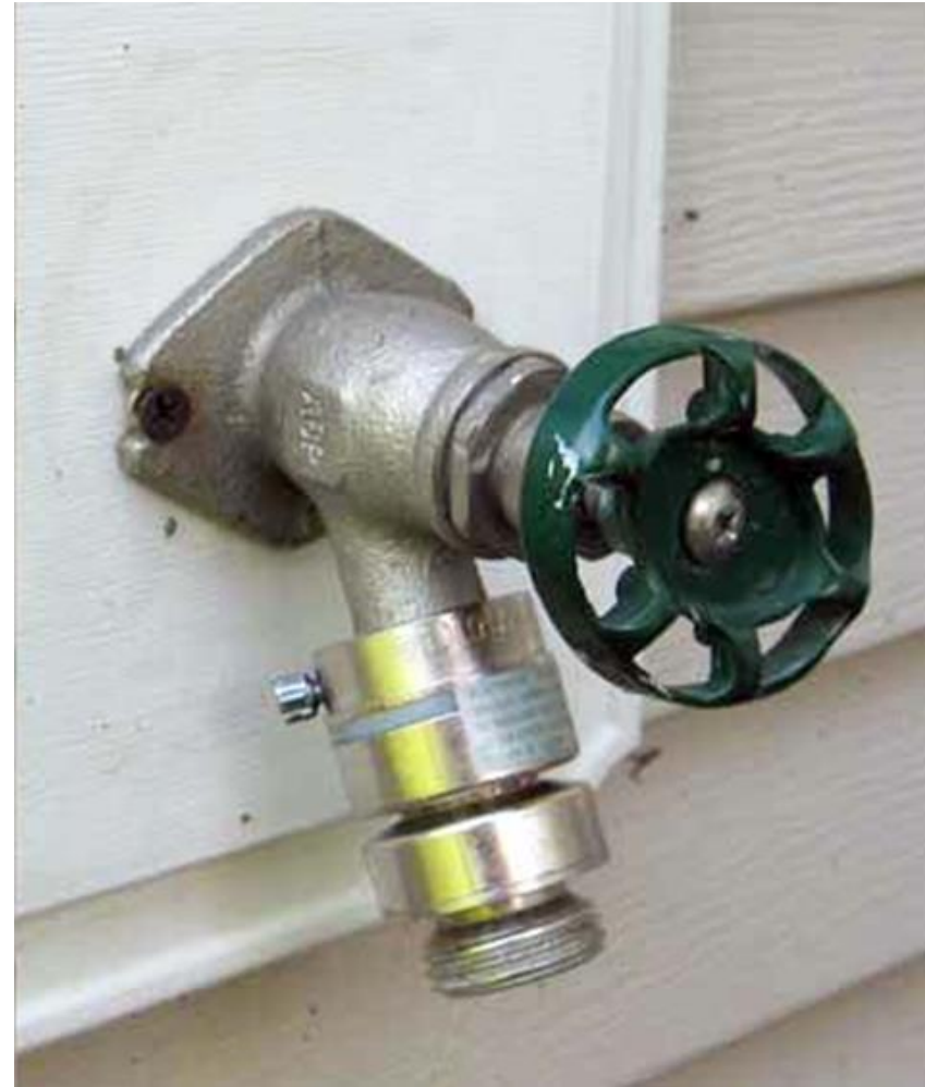
Vacuum breaker installed
