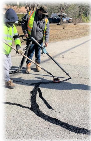
Crack Sealing on Jellison
